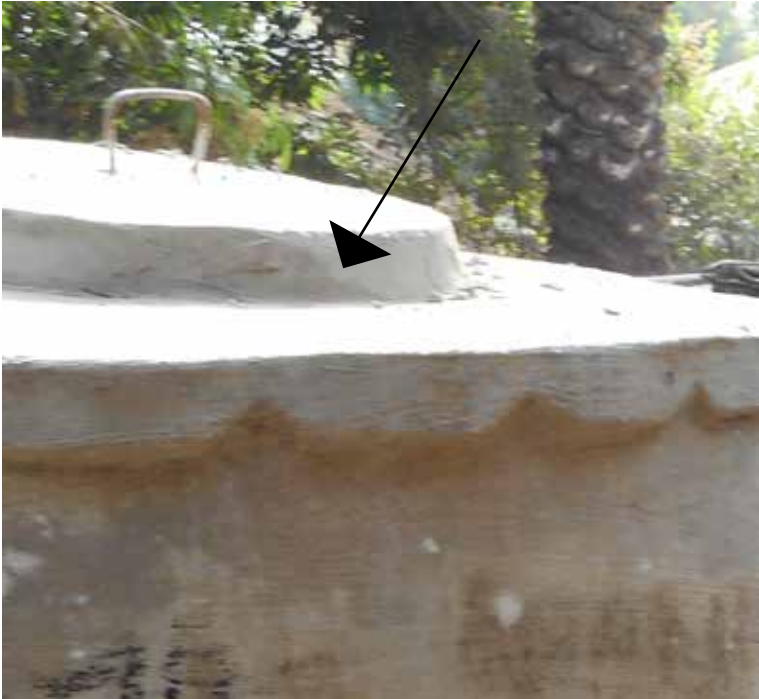
You can seal the lid with clay or soft cement to prevent that insects will enter the filled tank. 29
