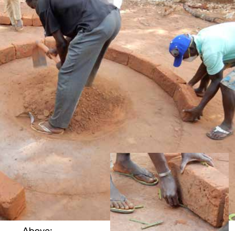
Above: adjust the clay blocks in the upright position.
