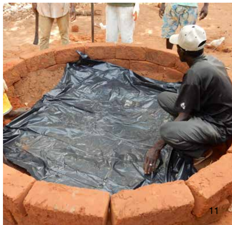
Below: place a plastic sheet to prevent the water from the mortar leaking away into the ground.
