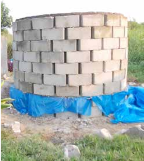
In DR Congo they sometimes use cement blocks for the mould
