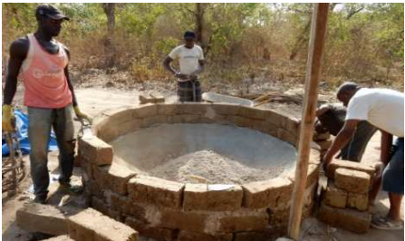
Construction of foundation. Twisting circle of steel wire for roof. Coordinators Paul and Kees watching the work
