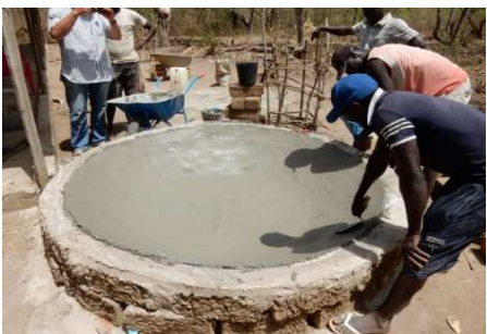
Construction of foundation. Twisting circle of steel wire for roof. Coordinators Paul and Kees watching the work
