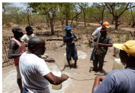
Construction of foundation. Twisting circle of steel wire for roof. Coordinators Paul and Kees watching the work
