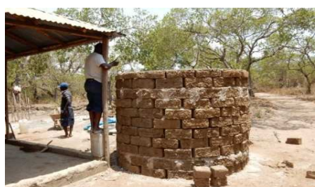
Construction of foundation. Twisting circle of steel wire for roof. Coordinators Paul and Kees watching the work
