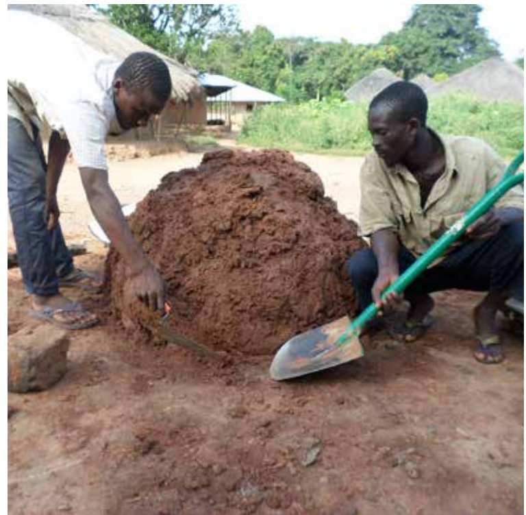
THE MIXTURE: 5 wheelbarrows of termite hill sand, a 50 kg bag of cow-dung, chopped rice straw in a 50 kg size bag.
