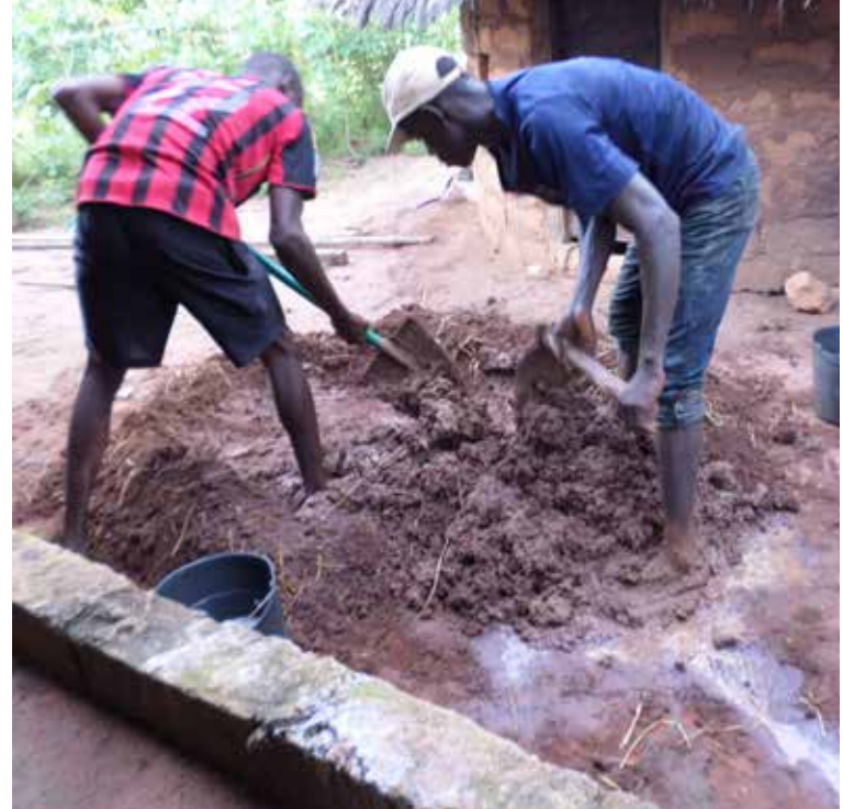
THE MIXTURE: 5 wheelbarrows of termite hill sand, a 50 kg bag of cow-dung, chopped rice straw in a 50 kg size bag.
