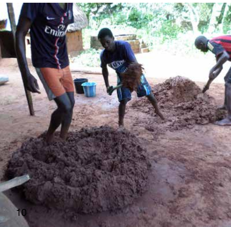
THE MIXTURE: 5 wheelbarrows of termite hill sand, a 50 kg bag of cow-dung, chopped rice straw in a 50 kg size bag.
