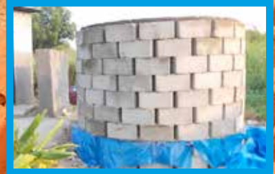
Cement blocks can be used, when clay blocks are not available.
