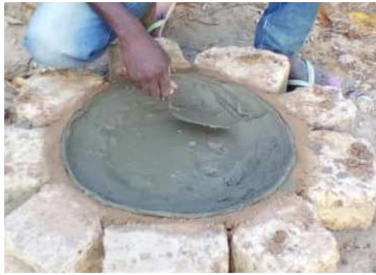
2+3 mould for the floor with mortar.
