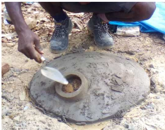
6. the roof is made on the ground, on a piece of paper of a cement bag.
