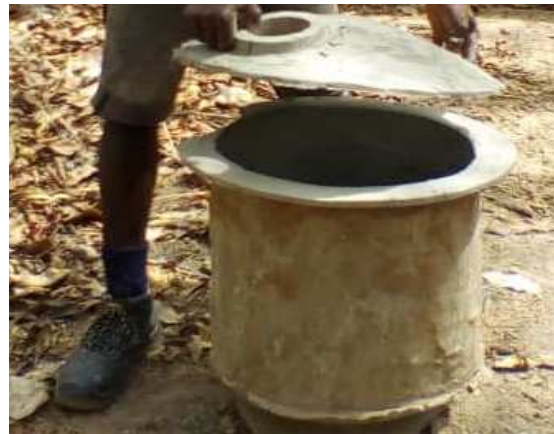
6. the roof is made on the ground, on a piece of paper of a cement bag.
