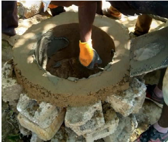
4. plastering 2 layers inside .....
