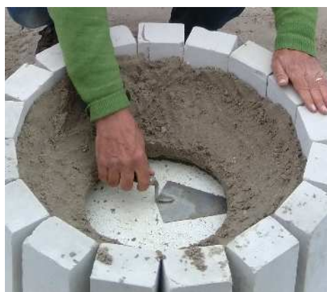
2 sand mould for the foot and the bottom
