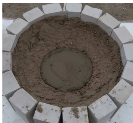
4 the foot has been poured
