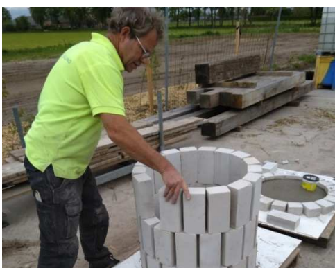
6. mould for the wall of blocks and damp sand. dark sand sticks better.
