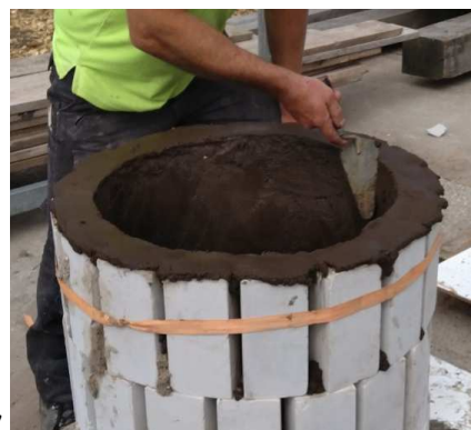
6. mould for the wall of blocks and damp sand. dark sand sticks better.
