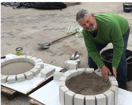
1. left: sand mould for the roof
