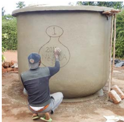
Figure 18.6 Finishing the outside. (Source: Author's own).
