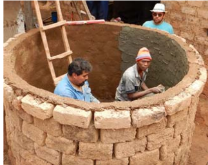
Figure 18.4 Plastering the inside of the mould. (Source: Author's own).
