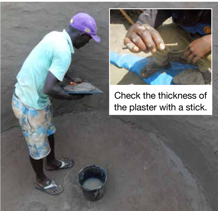
Above: mortar on wet sand. The mortar is curved over the edge of the mould. Below: apply a total of 4 layers of mortar during day 2, 3 and 4.
