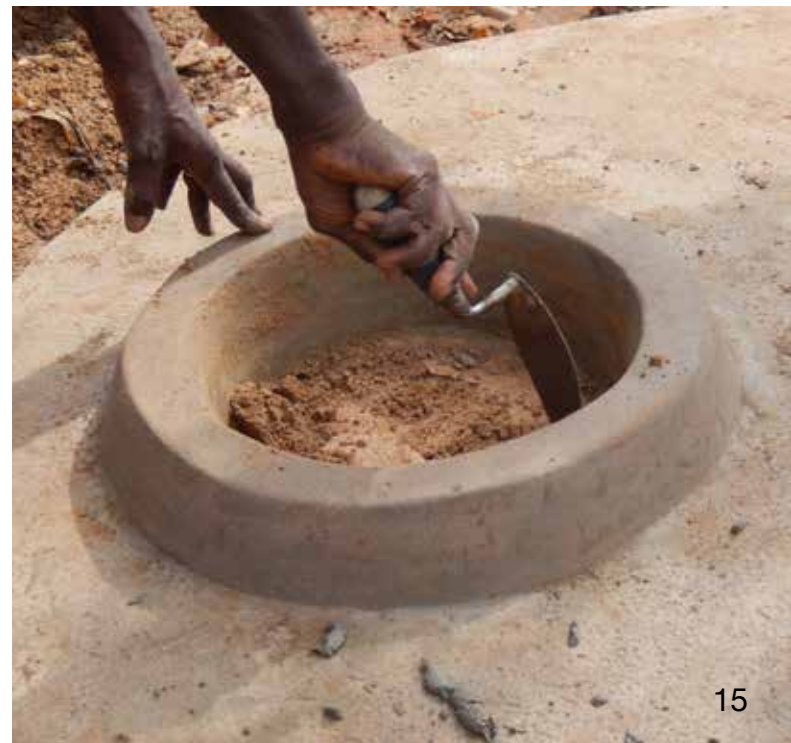
Above: the roof is reinforced with 4 circles of twisted steel wire of binding wire. Below: the construction of the manhole.
