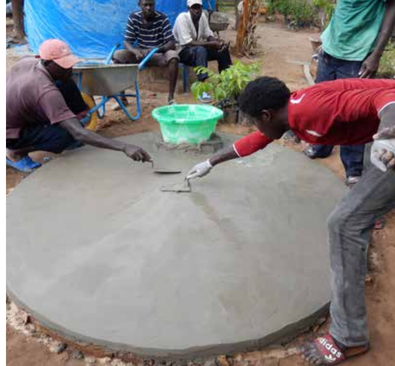
Above: the roof is reinforced with 4 circles of twisted steel wire of binding wire. Below: the construction of the manhole.
