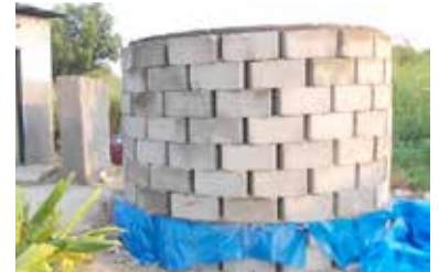
Cement blocks can be used, when clay blocks are not available.
