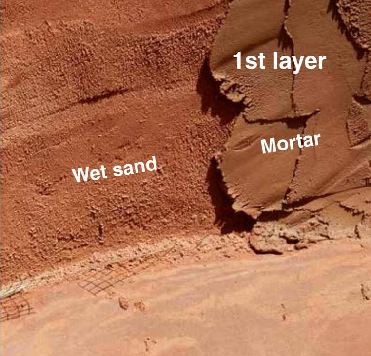
Above: mortar on wet sand. The mortar is curved over the edge of the mould. Below: apply a total of 4 layers of mortar during day 2, 3 and 4.
