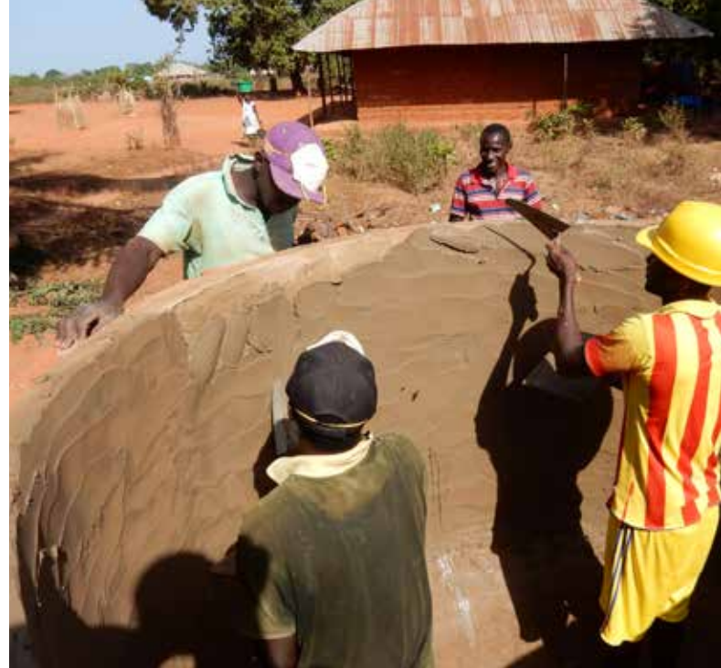
Above: mortar on wet sand. The mortar is curved over the edge of the mould. Below: apply a total of 4 layers of mortar during day 2, 3 and 4.
