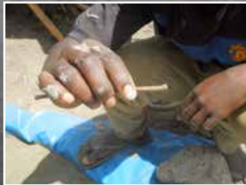
Check the thickness of the plaster with a stick.
