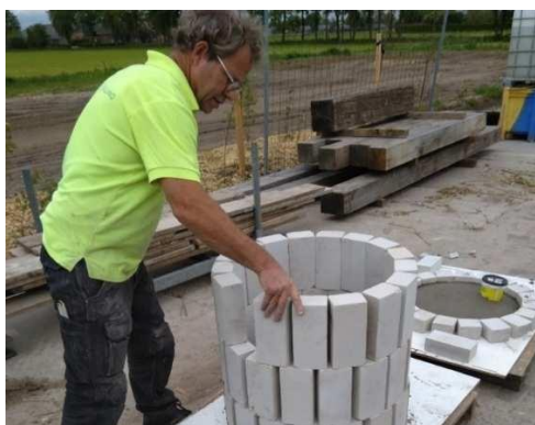
6. the form for the wall of blocks and moist sand.
