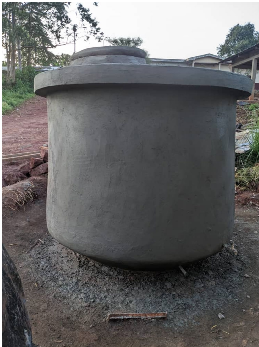
Fig. 3 Photograph of an Akerman Calabash with a capacity of 5,000 L ( 5 \text{ m}^3 ) in Feutap, Bangangté (Cameroon). A Calabash cistern collects and stores rainwater effectively while being cost-efficient and durable for rural settings. Photo taken by Vanick Fanseu (July 2024)
